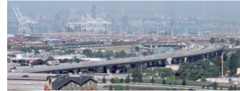
OpenSees project in CE at Berkeley looks at this section of 880, among others
