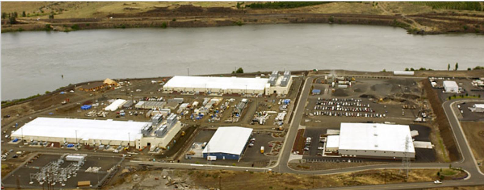
Google data centers in The Dalles, Oregon
