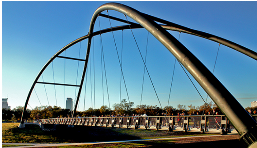
Figure 6: Bill Coats Bridge in the Hermann Park in Houston, Texas [7].
